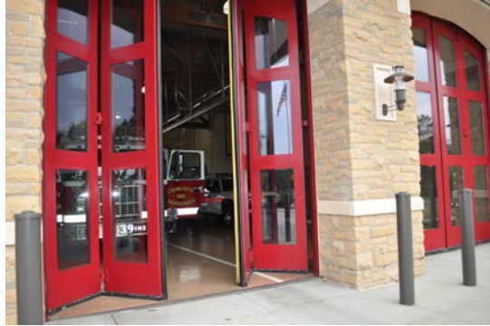
Figure 4.12 — Another exterior view of a folding bay door.
