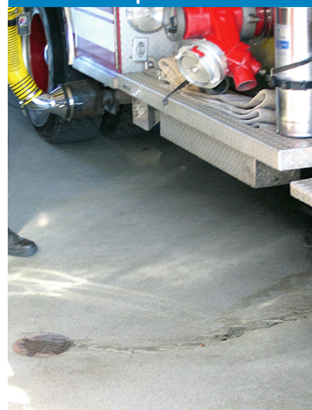
Figure 7.8 — Improper placement of apparatus floor drains create wet spots that will cause slips and falls.
