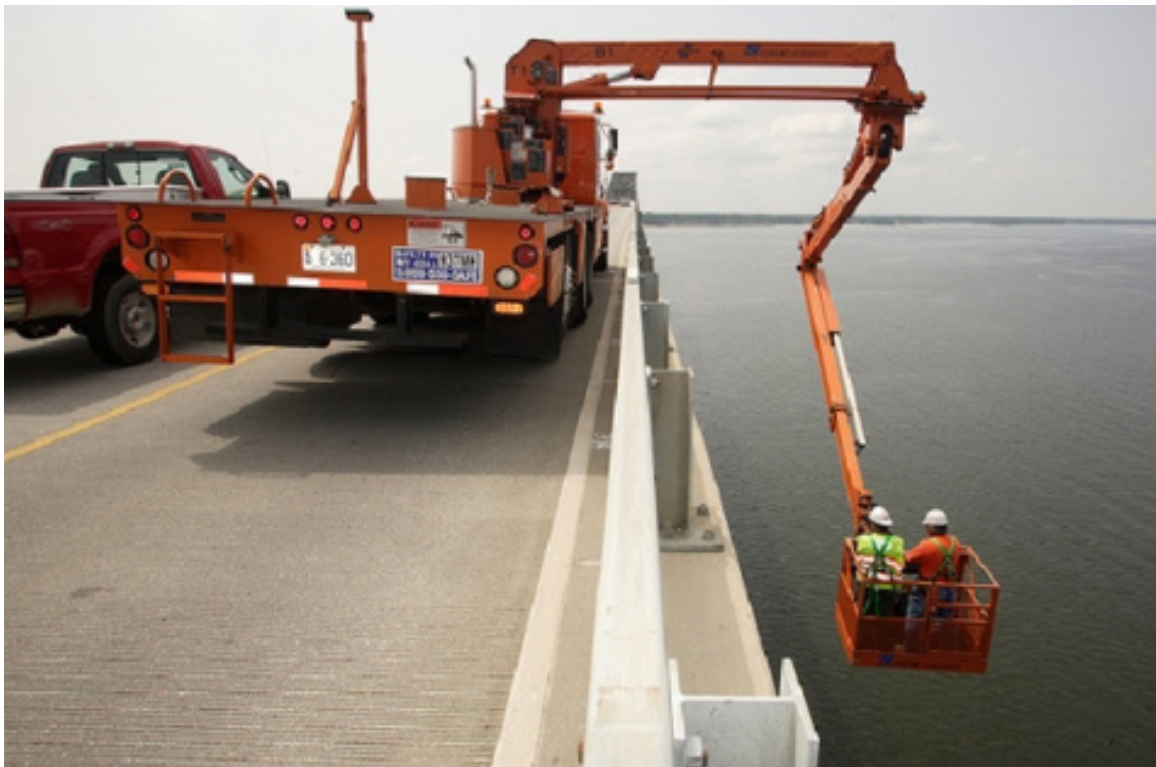
Figure 3. Example of Workers Conducting Bridge Maintenance from a Snooper Carriage (Reproduced from (Chen, 2014)) 7
